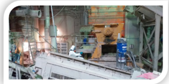
Dismantling conveyor system, waste preparation line
